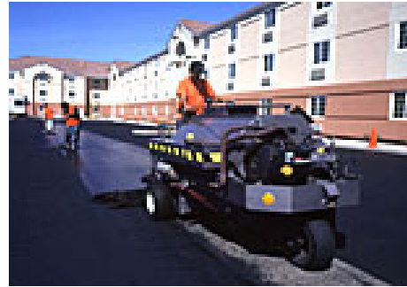
Seal Coating Application
